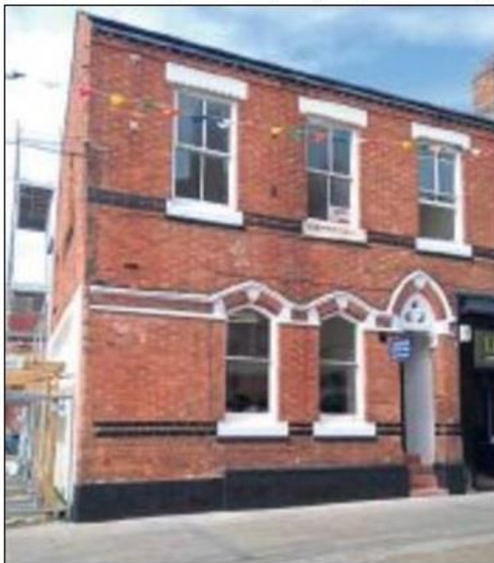
Three of the five suites of offices in the Yards Business Centre were pre-let before refurbishment was even complete.
